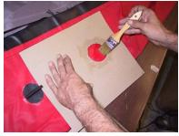
**4.** Apply the patch as shown on illustration. Note: **The loop in each patch must be horizontal.** Move the template so the top edge lines up with the seam and the side that is 7.5 inches (19 cm) from the hole touches the patch you just installed. Repeat the process with the next patch. Continue until you get to the end of the canoe skin.
